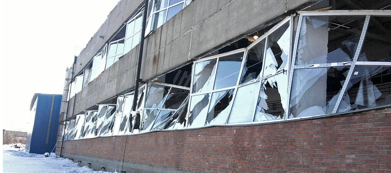
Factory wall after it was hit by the blast wave. Image credit: Константин Кудинов
